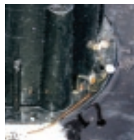
Excessive nailing
